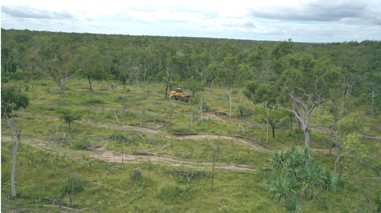
Figure 3. A loader pushing access tracks through debris.
